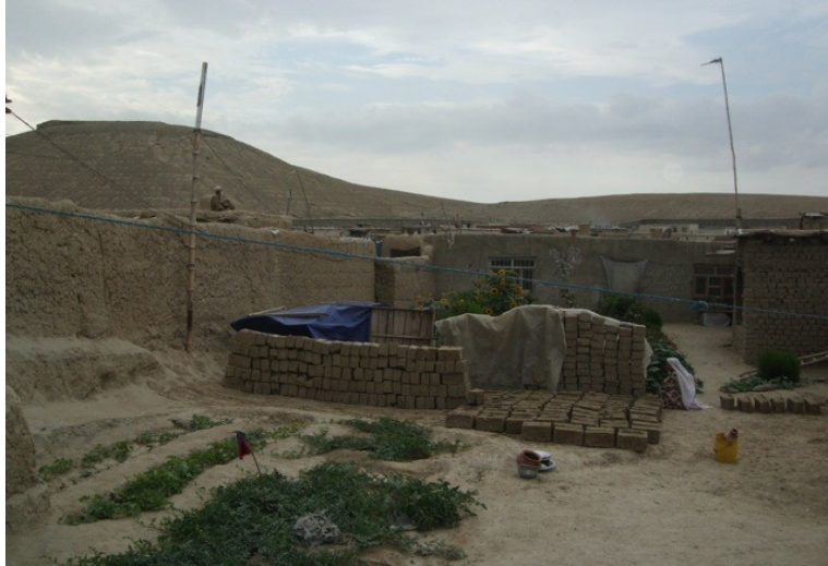
Photo 3: House under construction, Pole Charkhi informal settlement (Kabul)
