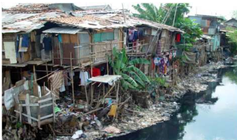
Figure 4: An urban community built on a water body in Cambodia
