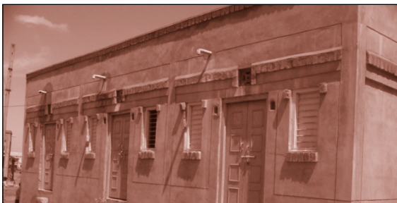
Contractor-built houses in Gujarat
