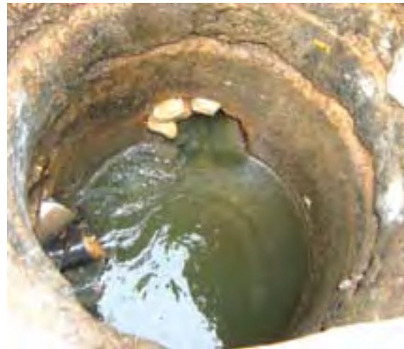
Open manhole for sewage and rain water disposal in Baraksat
