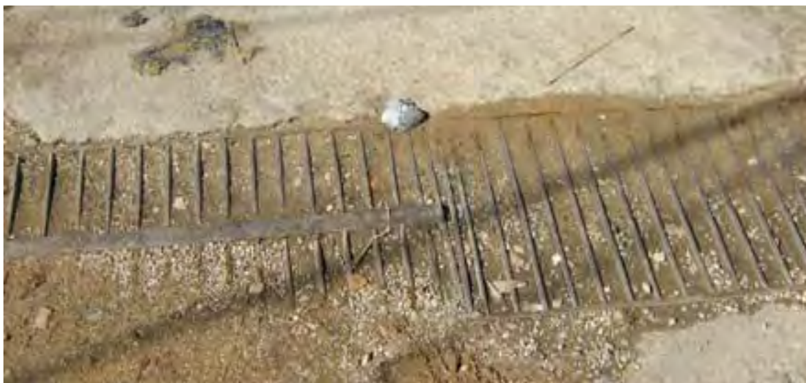
One water drain (blocked) was installed by UNRWA at the entrance to Fadlo Wakim
