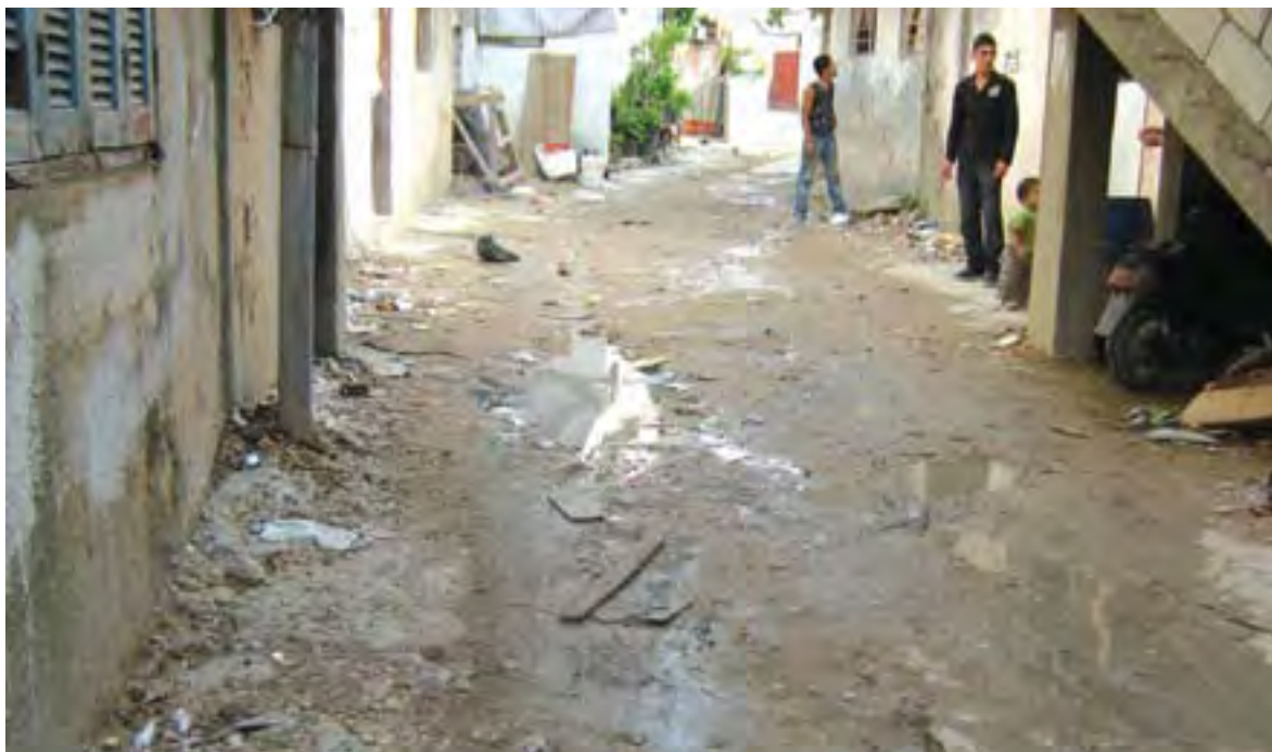
Unpaved internal roads in Baraksat
