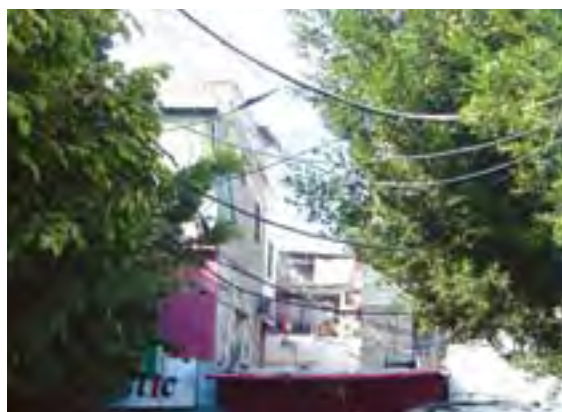
Water provision in Hay el Sohoun is compromised by the ad-hoc electricity connections (Note partially repaired cables)
