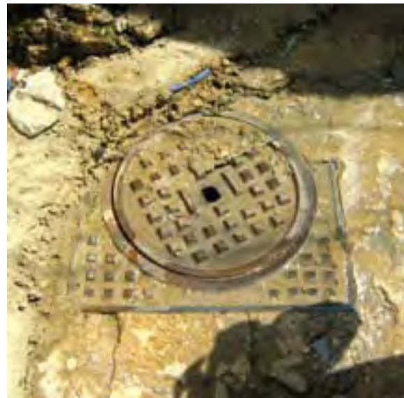
Manholes installed by UNICEF in Mouhajarin
