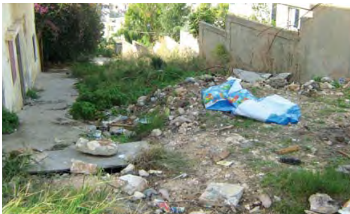
In addition to rehabilitation, roads in Jabal el Halib need a drainage system that suits the strong sloping of the AA
