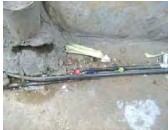
Above ground house connections installed by dwellers in Tawari to access water
