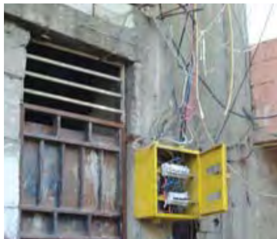
Electricity meters initially installed by EDL were replaced with direct connections to electric distribution boards by the SC in Hay el Sohoun
