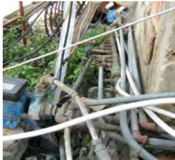
Direct implementation of water networks by dwellers in the AA of Jabal el Halib around Ain el Helwe Camp
