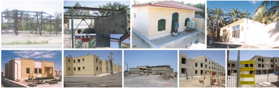
Fig. 5 Reconstruction of Bam in terms of individual dwellings and apartment buildings
