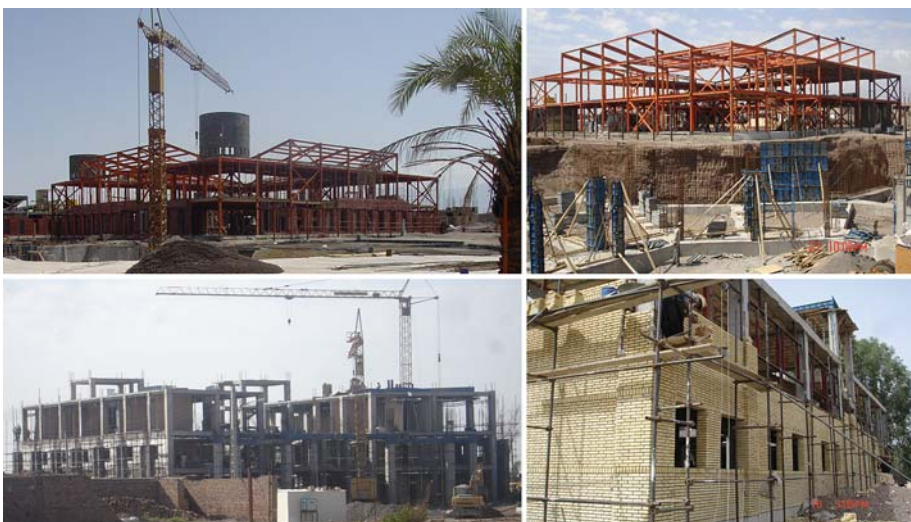
Fig. 9 Reconstruction of Bam government building complexes
