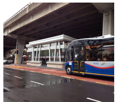
MyCiTi bus and feeder station, Gardens
