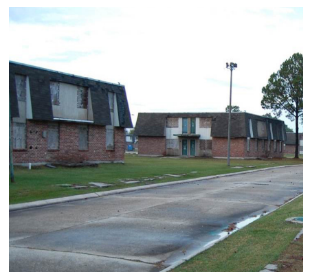
Original homes of the first Vietnamese migrants in New Orleans (damaged by Hurricane Katrina)
