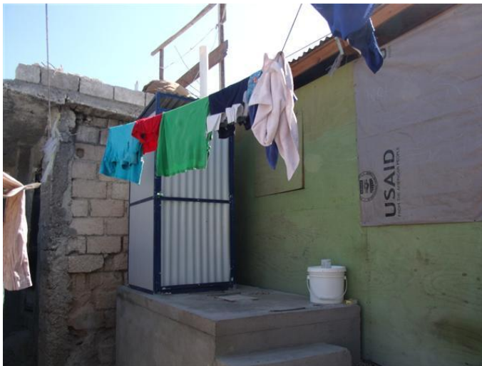
A new CRS urban double vault latrine in Solino, shared among 3 families.
