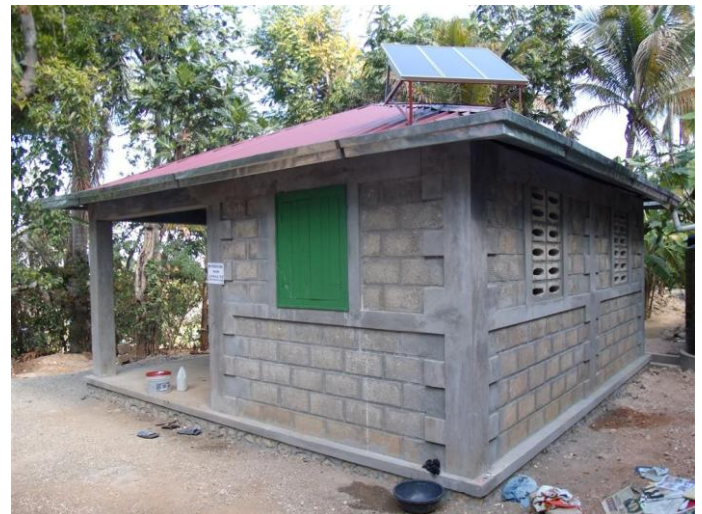
A Caritas Switzerland 3 room earthquake and hurricane resistant house. The solar panel is only on this house for demonstration purposes, but all houses are wired for electricity.
