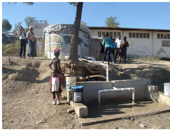
A former CRS camp water system supplied by water trucks (now paid for by the beneficiaries themselves).
