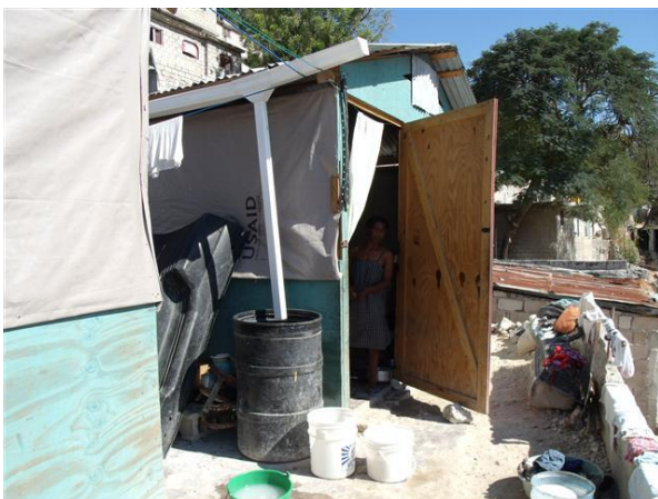
Rainwater gutter and downpipe. People usually keep the 30 gallon tank inside to prevent it from being stolen.
