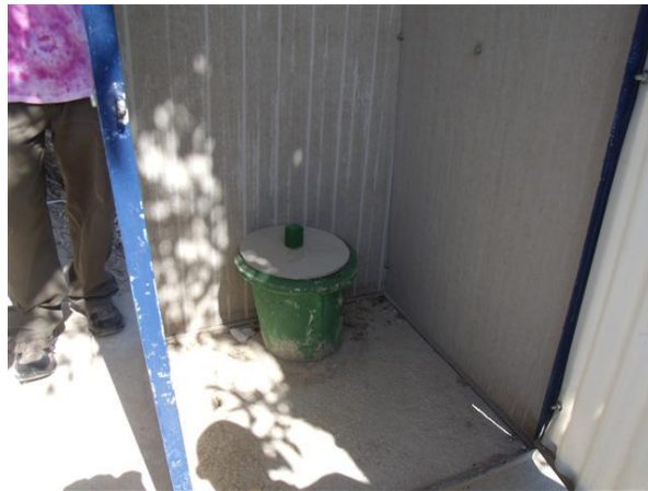
The inside of a latrine with a concrete seat and a seat cover. Sometimes there are gaps between the cover and the seat, allowing flies to pass through.
