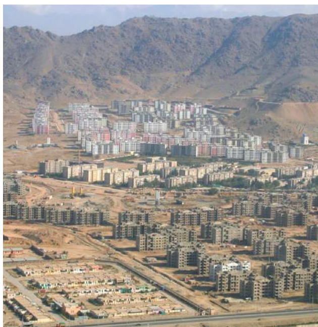
Apartments under construction, Kabul
