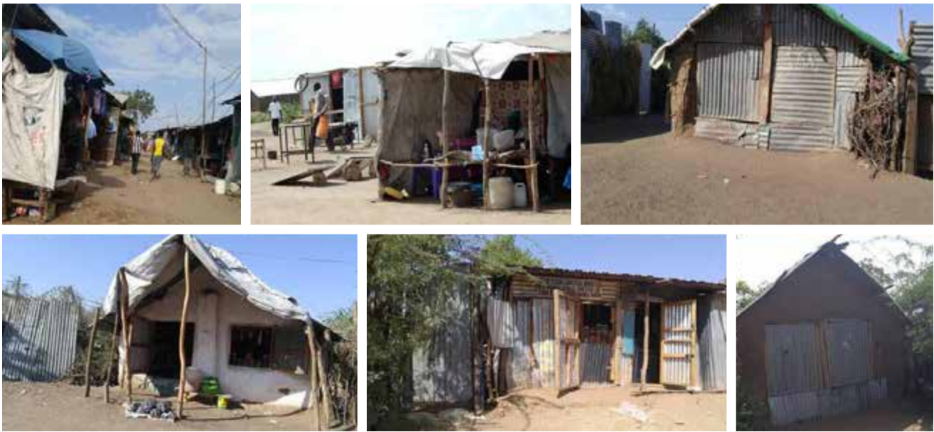
Figure 75: Variations in Material Used for Commercial Extensions in Kakuma Camp
