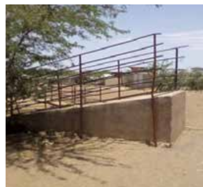
Livestock loading zone
