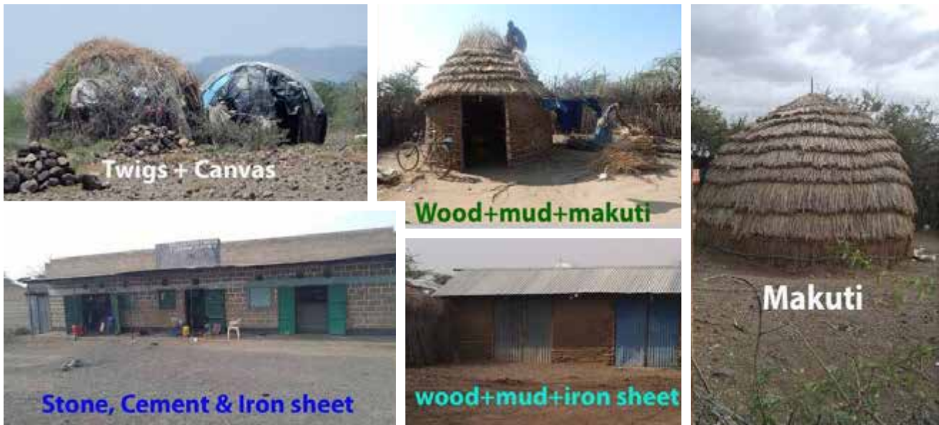
Figure 52: Varying Walling and Roofing Materials in Kalobeyei Host Community Areas
