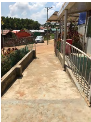
Camp 15 : Access ramp
