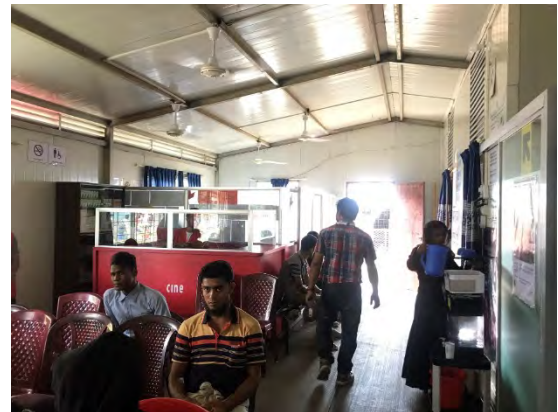
Interior (no visible bracings)
