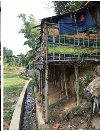
Shelters on stilts
