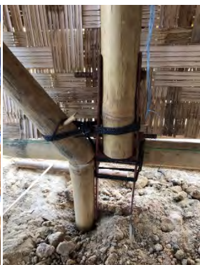
Detail of bamboo footing
