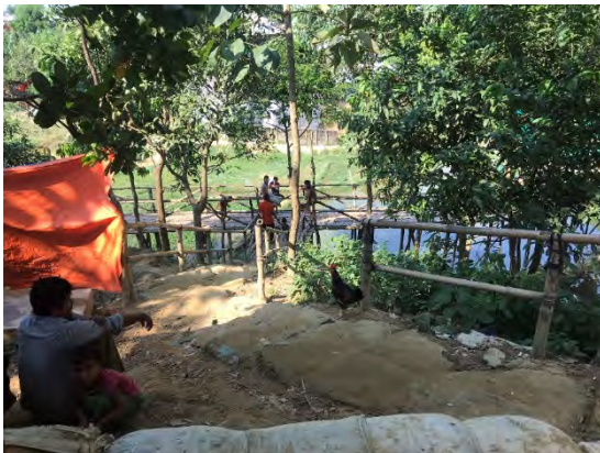
Main access entrance (bridge and stairs)
