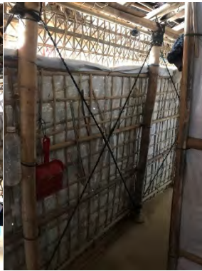
Upper wall ventilation and bracing details
