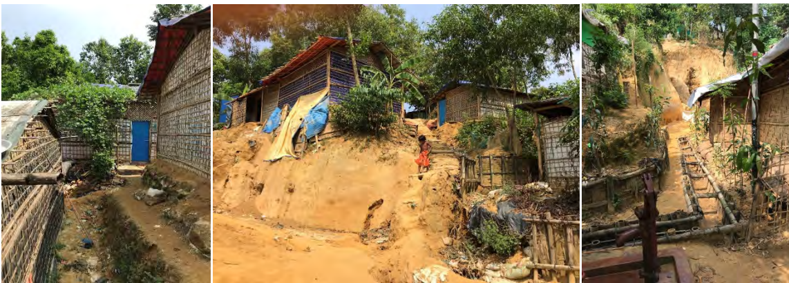
Camp 19: no drainage
