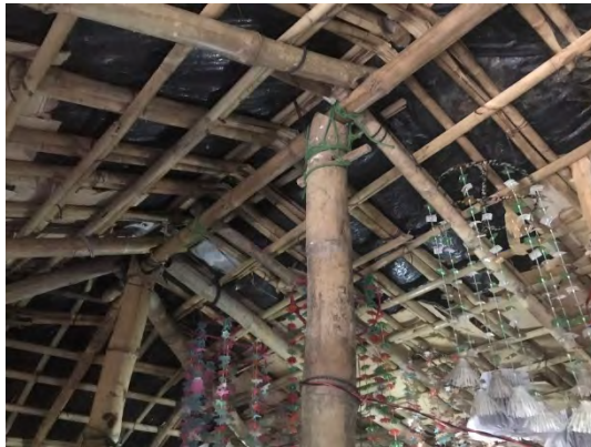
Bamboo connections
