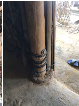
Medair's personal developed bamboo footing
