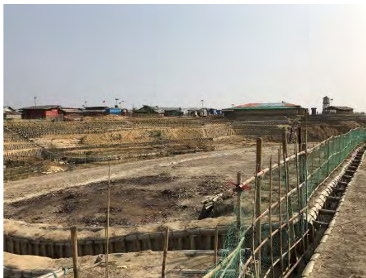
Site development: soil stabilisation & drainage
