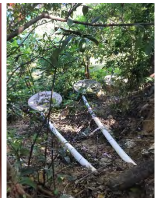
Toilet pits close to the river
