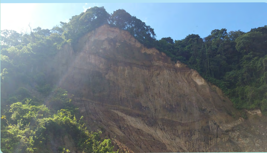
The slope of the cliff above El Cambray Dos after the landslide. Photo credit: Leah Campbell, ALNAP.
