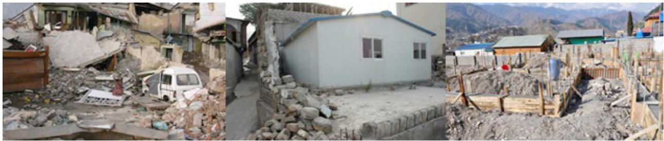
L: earthquake damage in urban areas in 2005 following the Kashmir earthquake. Centre: temporary shelter still in use, and occupying plot, in 2010. Right: urban housing reconstruction underway in 2018 with no technical assistance. All photos taken from keynote speech, 'What went well? What could have gone better? Learning from recovery experience in Nepal and Pakistan', from June 2018 Risk2Resilience conference.
