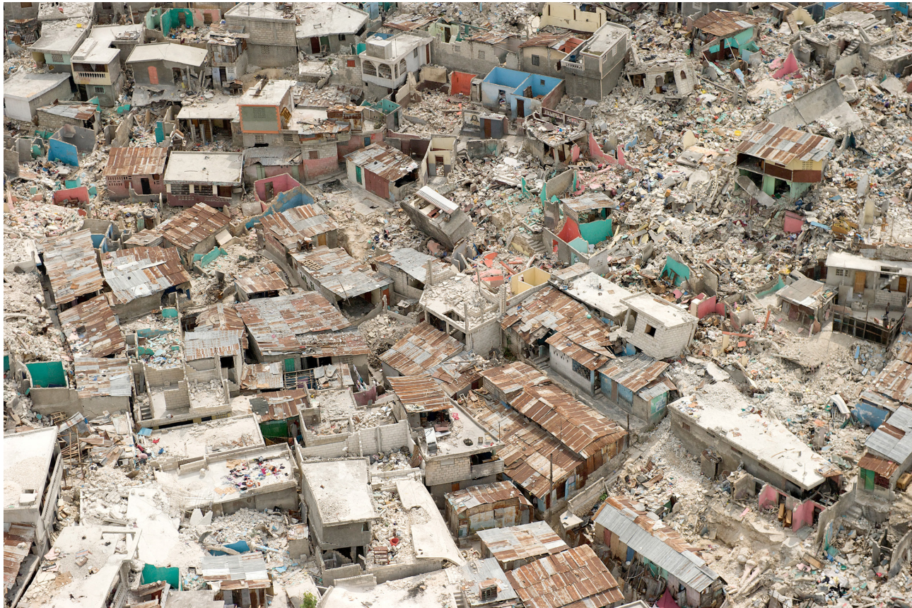
An aerial view of earthquake damage to housing in Port-au-Prince.
