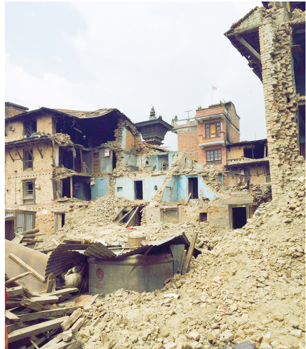
Earthquake damage in Bungamati in June 2015. Photo credit: Jake Zarins / Habitat for Humanity.
