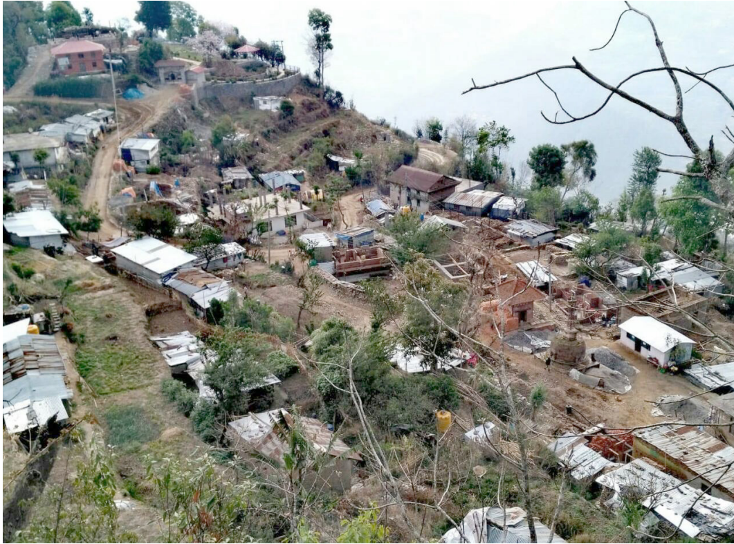
View of the old core, urban area in Bhimeswhor Municipality, Dolakha. Photo Credit: NSET.
