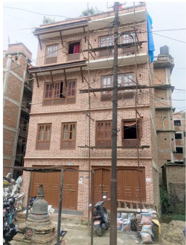
Newly constructed house under Pilachhen Reconstruction and Tourism Project.
