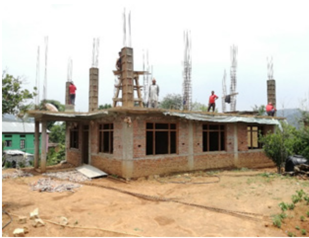
Housing Typology: Reinforced Cement Concrete Framed Building (RCC)
