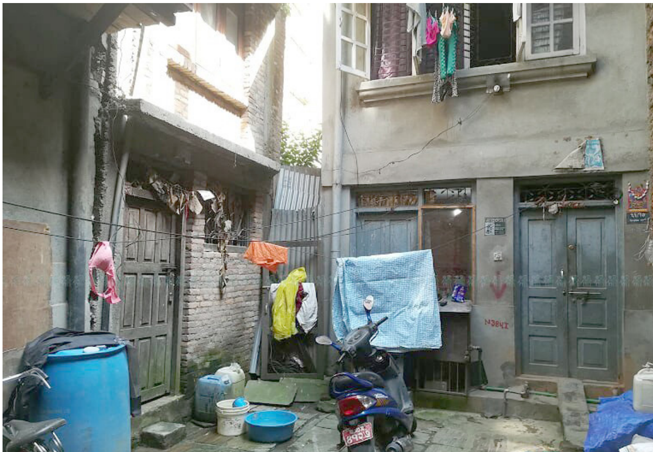
Part of the area in Dambochowk where house pooling will be implemented by a group of 54 households.
