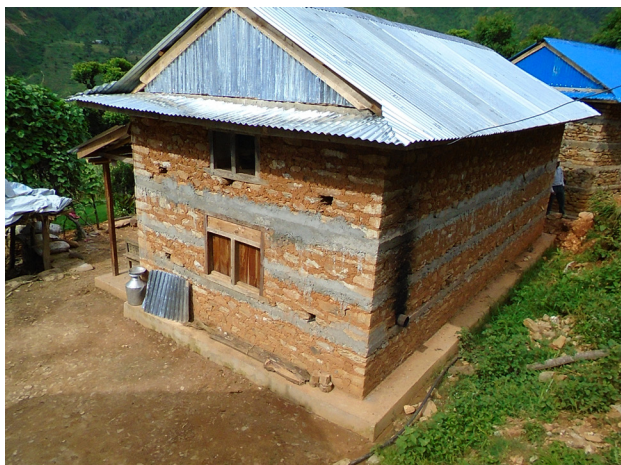
Housing Typology: Stone and Mud Mortar Masonry Location: Ramechhap, Ramechhap Municipality, Ward No. 9 RC bands have been used and a light gable has been constructed from CGI.
