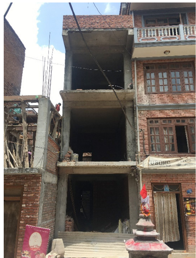
Housing Typology: Reinforced Cement Concrete Framed Building (RCC)
