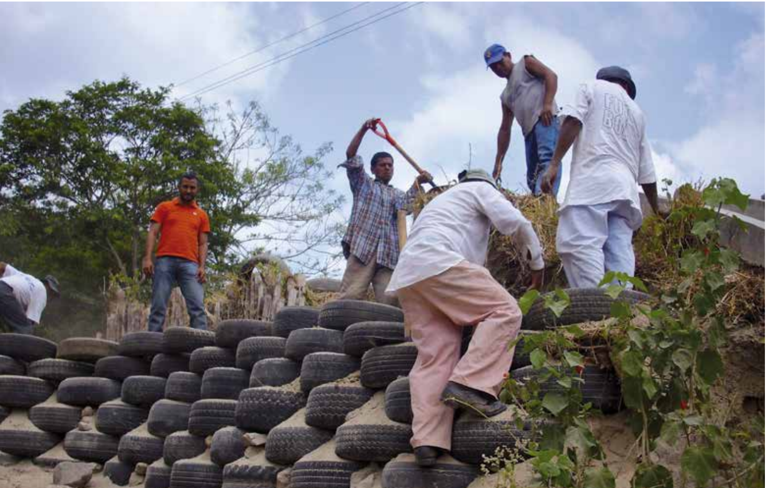
In Guatemala, scrap tyres are used to reinforce erosion-vulnerable roads and embankments. This low-cost risk reduction measure not only protects local infrastructure investments from erosion, but also contributes to solid waste management through reuse and recycling (Photo: UNISDR/Margarita Villalobos).
