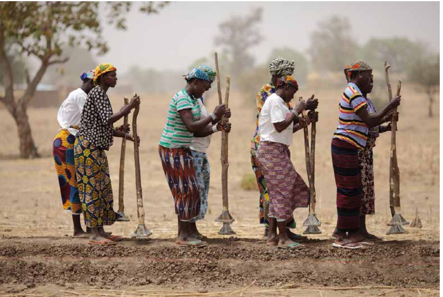
Africa yet again suffered from major droughts in 2012. In order to increase their resilience, women in Burkina Faso are building a dyke to contain rain water for cultivation (Photo: European Commission DG ECHO).
