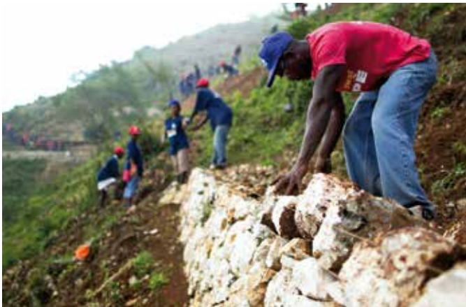
Residents in Haiti building rock walls and planting vegetation as ways to save arable land and avoid flooding in lower areas (UN Photo/Logan Abassi).
