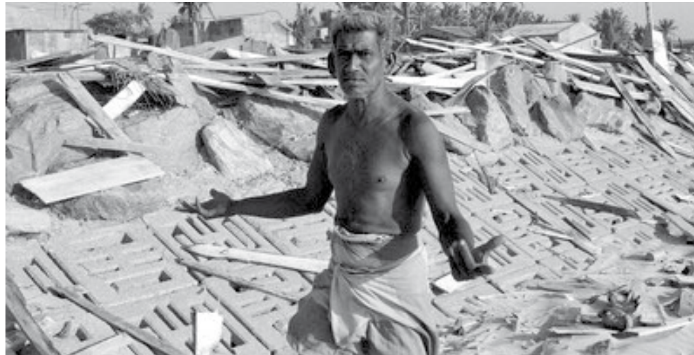
Destruction in Sri Lanka. The tsunami caused billions of dollars damage in many Indian ocean nations. Photo © UN
